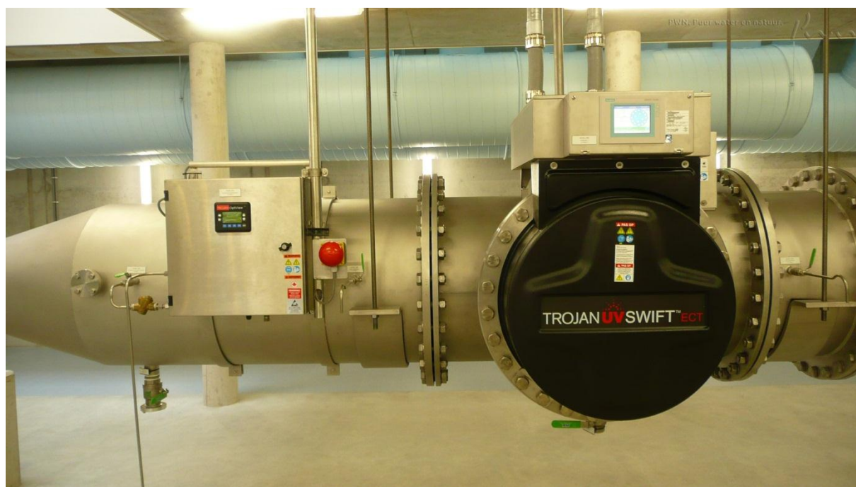
Figure 2.16: The polychromatic TrojanUVSwift™ECT system with cross-flow lamp configuration (PWN, 2012)
